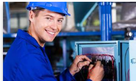
Service de maintenance Maintenance Service
